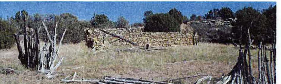
5LA.11794 Remains of loafing shed, barn, and corral
