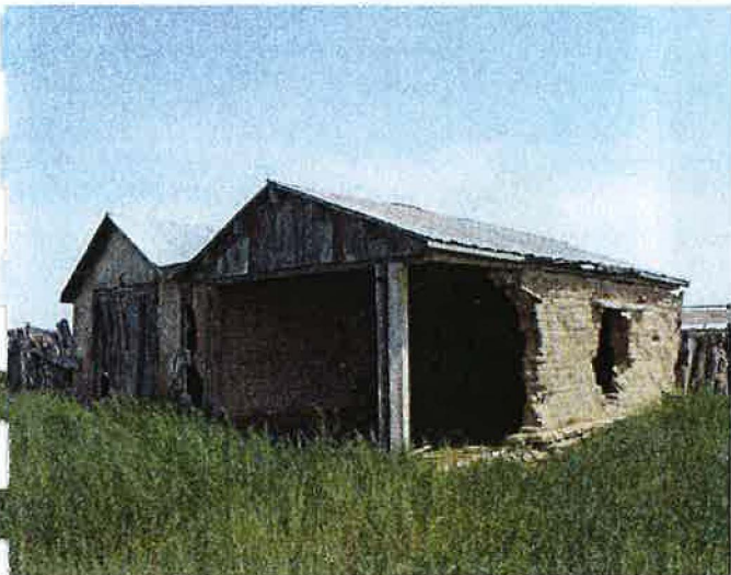
5LA.11897 Adobe block construction
