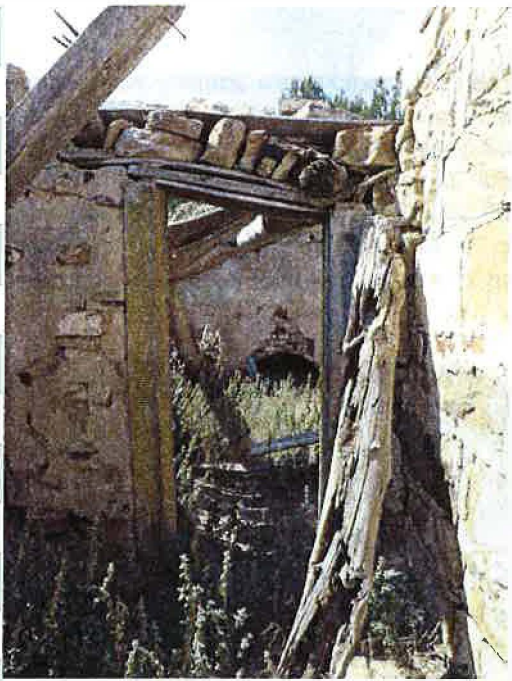
5LA.11635 Interior of dwelling
