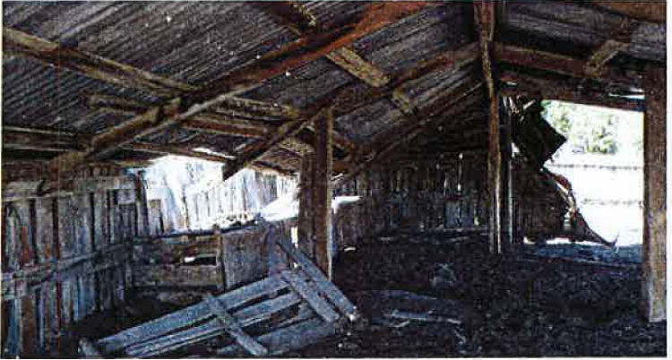
5LA.11717. Lambing shed
