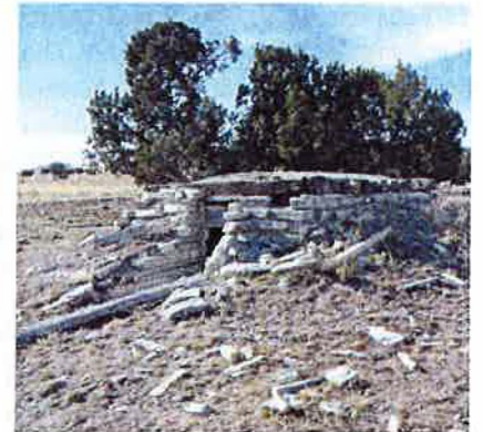
5LA.11895 Dugout constructed with stone and a roof of railroad ties
