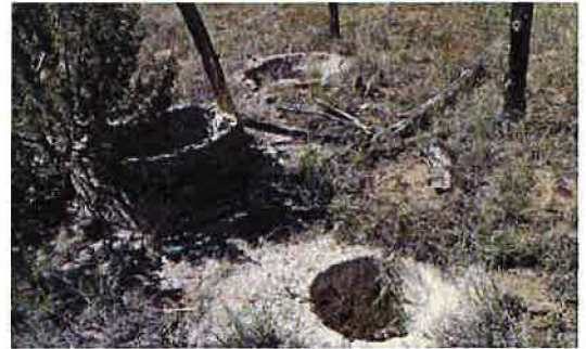
5LA.11759 Cistern with filters
