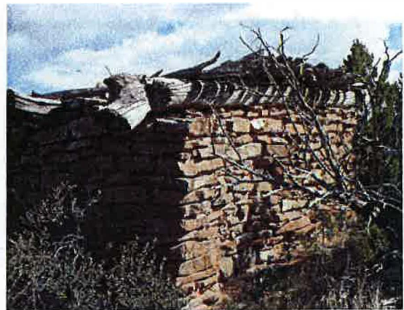
5LA.11761 Viga and latia roof construction
