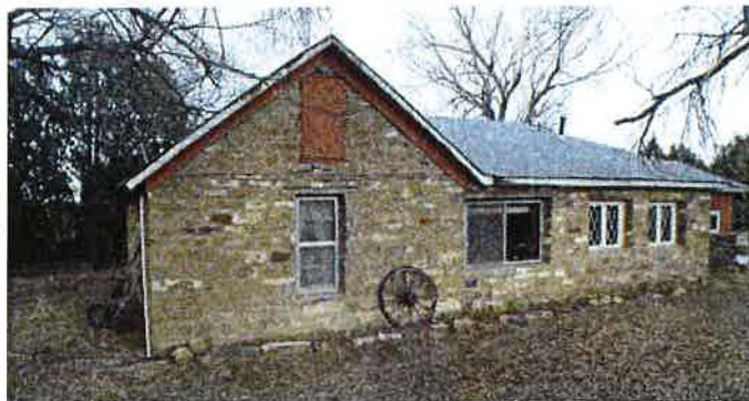
5LA.11872 A stone house dating to the 1910s is part of a modern ranch headquarters
