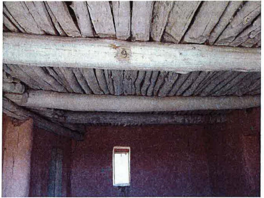
5LA.11736 Interior view of viga and latia roof construction
