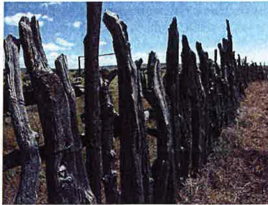
5LA.11582-4 A corral constructed of closely placed unfinished logs sunk vertically into the ground and held in place with wire tying them to a horizontal log
