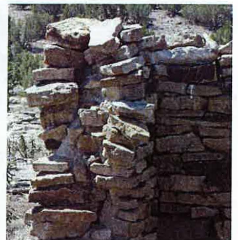
5LA.11676 Double stone wall construction
