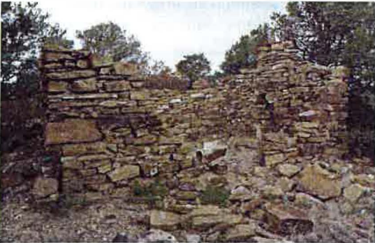
5LA.11840 Building of mostly fieldstone
