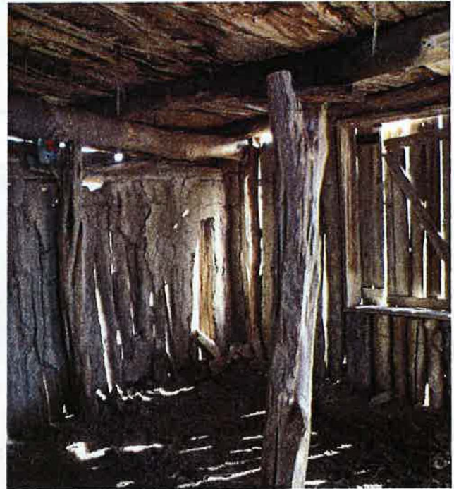
5LA.11736 Interior of jacal structure
