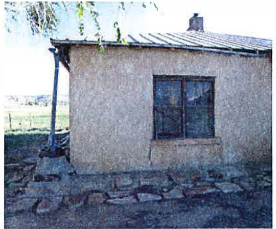
5OT.1104 Corner cistern
