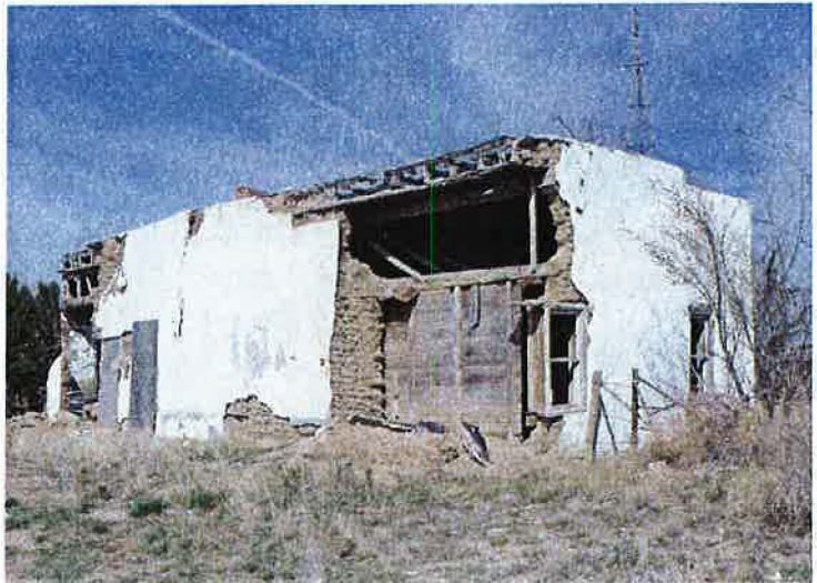
5LA.11913 Adobe block construction was also used for commercial buildings such as the Tyrone Store.
