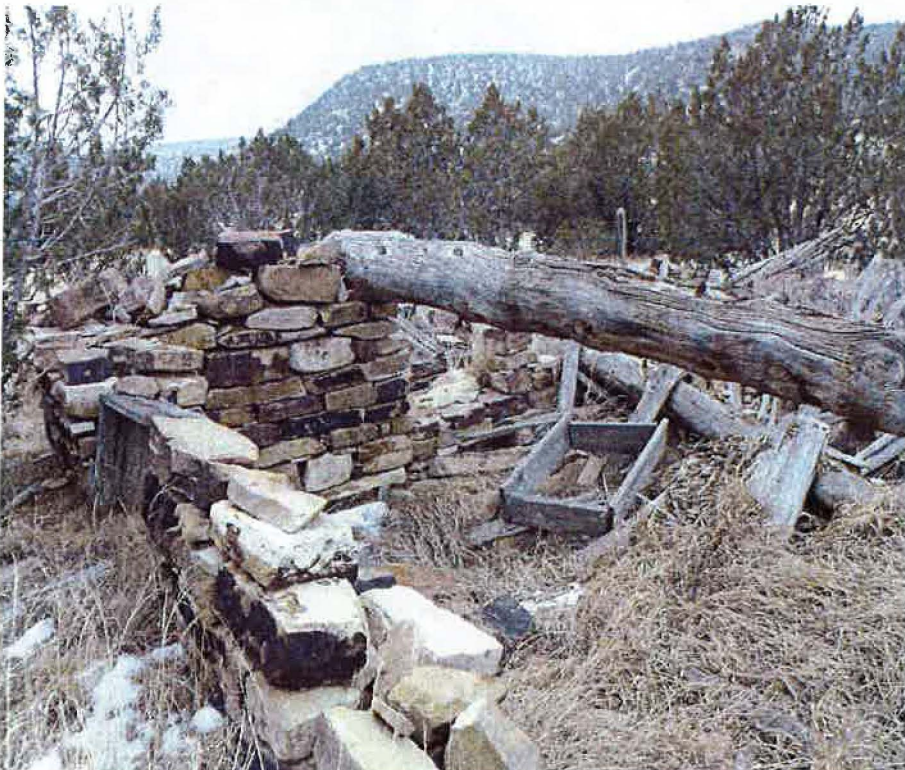
5LA.11880 Homestead showing roof beam and window framing
