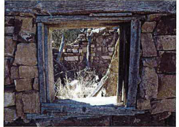
5LA.11781 Window frame of milled lumber
