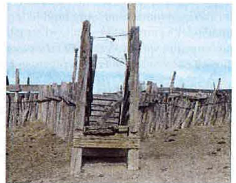
5LA.11897 Loading ramp
