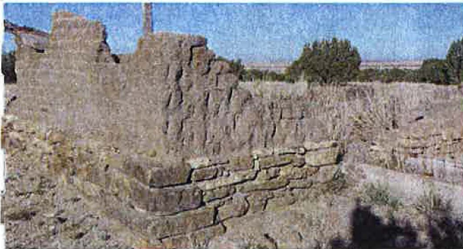
5LA.11791 Once exposed to moisture, adobe blocks rapidly deteriorate. Surviving uncovered adobe walls like one were rare. The all stone foundation has likely helped to preserve it
