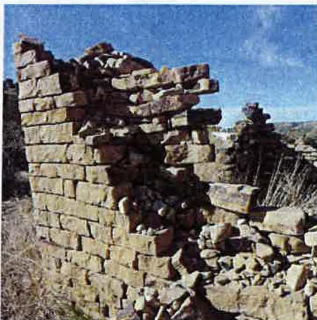
5OT.1105 Double stone wall construction
