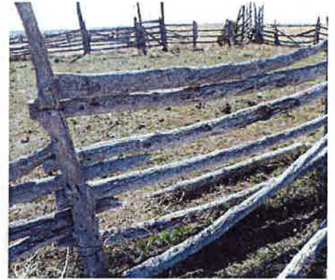
5LA.11836 A corral composed of horizontally placed logs slid between paired upright posts
