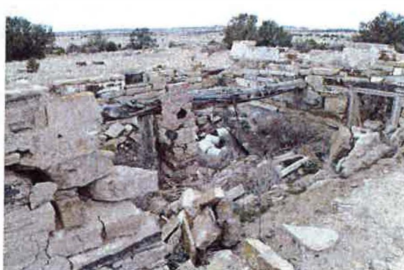
5LA.11895 Dugout constructed with stone and a roof of railroad ties
