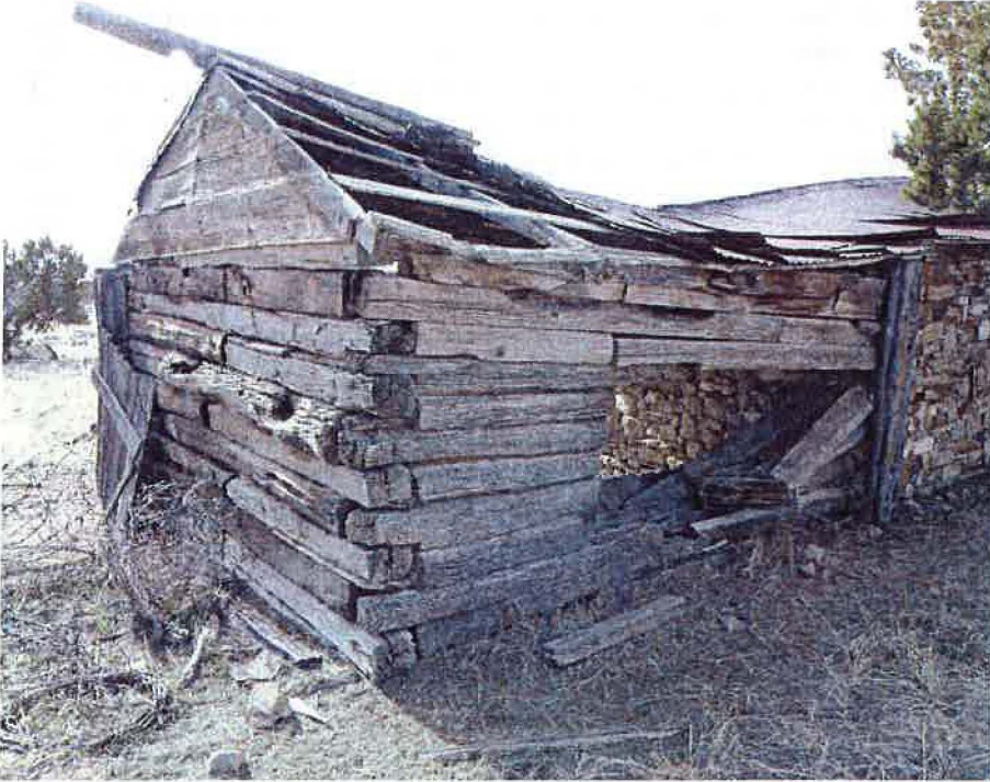
5OT.1172 Barn constructed with stone and railroad ties
