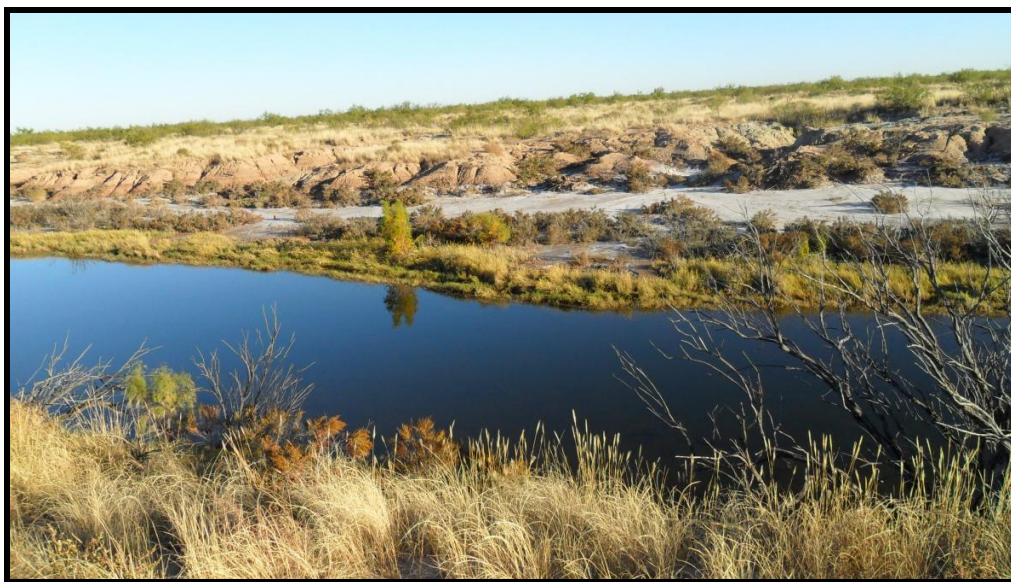
Looking at eastern side of Comanche War Trail embankment
