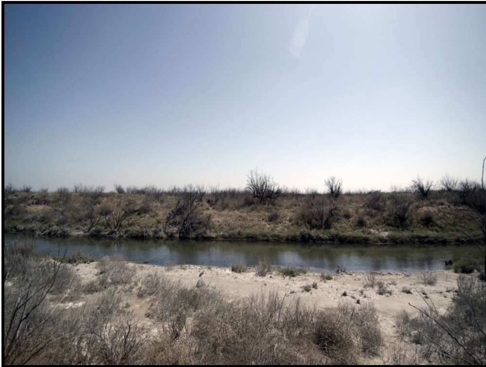
Looking at eastern side of later cattle crossing broken down embankment
