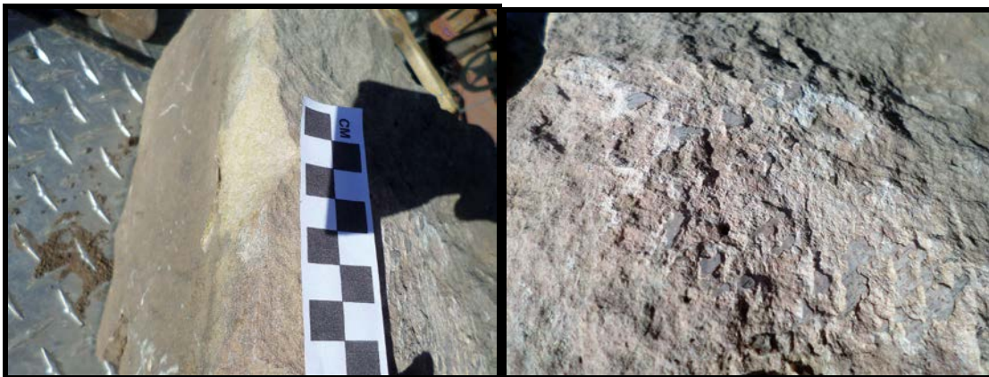
Mortar on side and top of large limestone block
