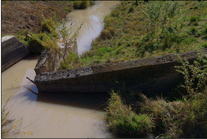
Figure 4.21: Ruin of a 1937 cement irrigation headgate placed in the 20th century Battle Creek ditch in the Lower Ravine.
