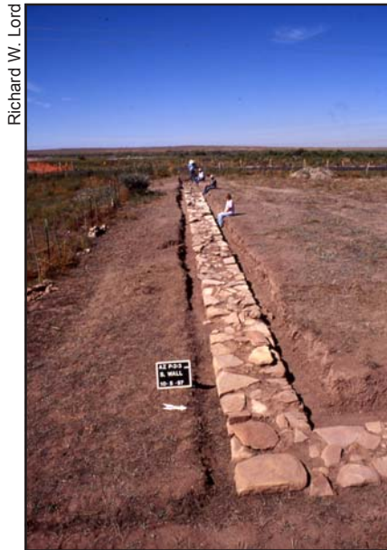
The southeast corner of the fort, looking down the length of the south wall, with Arizona Archaeological Society volunteers spaced every 20 feet.
