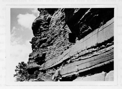
Fig. 10. Uncoursed, wet-laid masonry storage unit--42Sal813.
