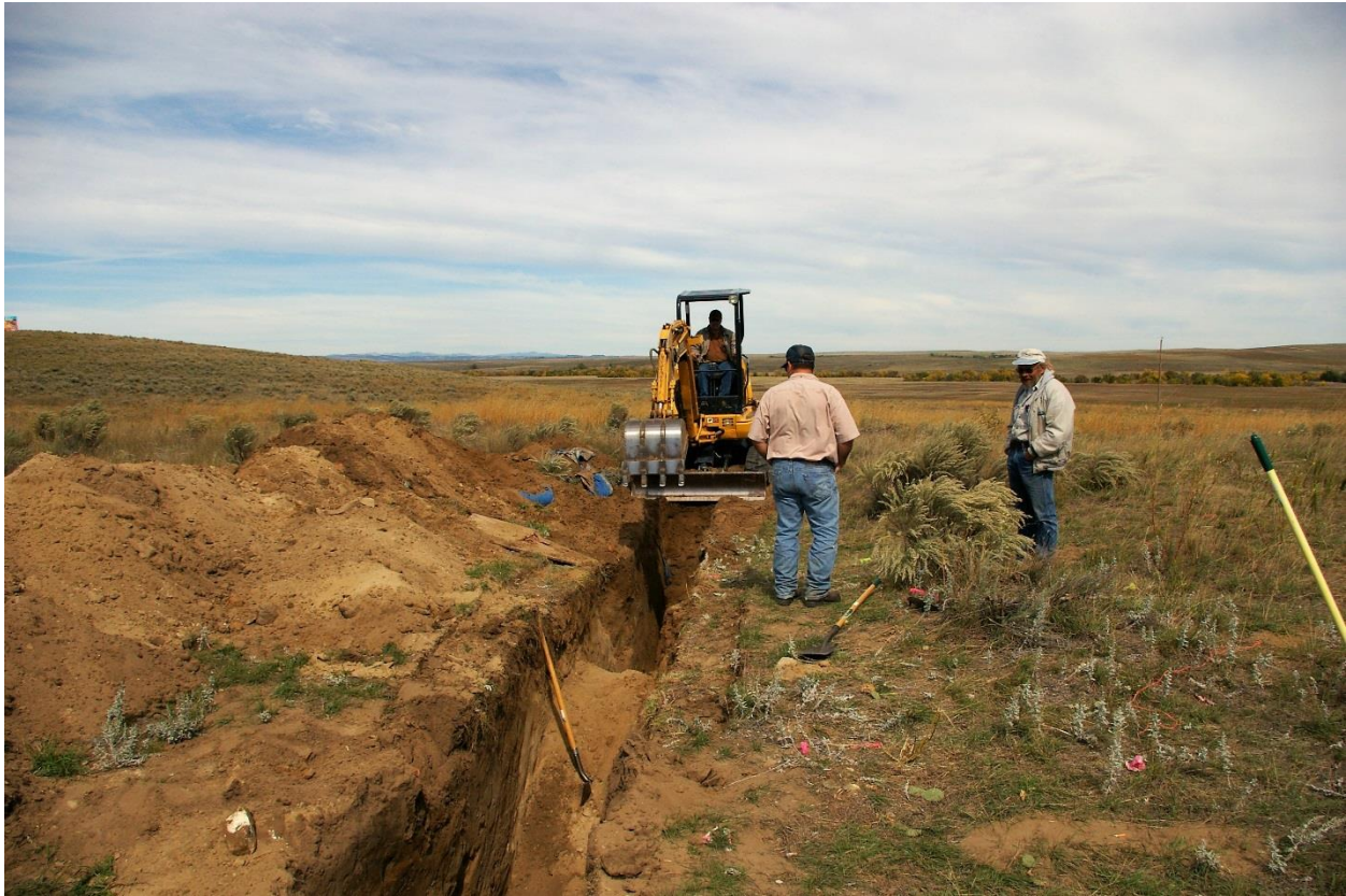
Figure 3. Digging a backhoe trench to facilitate geomorphic study of a site, 2006 (ARC photo).
