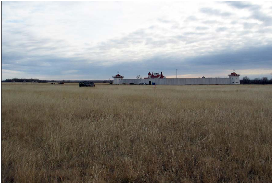
b) general view of Grid Area 8 (view to the southeast)
