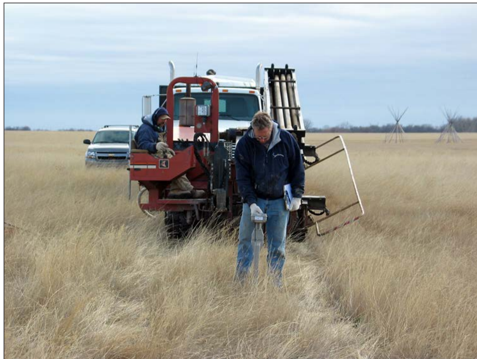
b) view of drilling operation in progress (view to the east)
