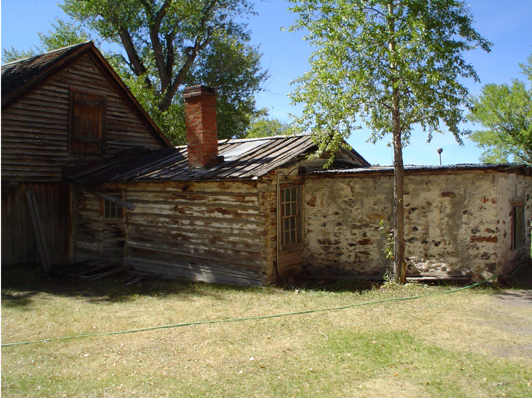
FIGURE 17. Rear view of the Finney House featuring several of the building additions the family added throughout the years. The building in the center is the original 1863 one-story log cabin with a low-pitched roof. In 1864 a one and a half-story gabled roof log structure was added to the front of the cabin. Unfortunately there is no construction date for the stone root cellar added to the rear of the building (Photo by author, 2007).
