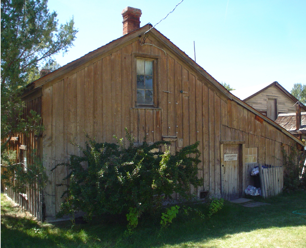
FIGURE 16. Rear view of the Dr. Byam House showing the 14'x20' shed added to the home in the nineteenth century (Photo by author, 2007).
