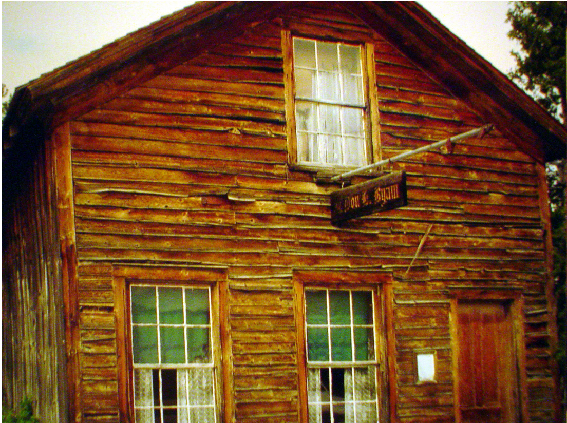
FIGURE 15. Front view of the Dr. Byam House. The Dr. Byam is architecturally classified as a false-front building of frame construction with a wooden shingle roof. When the house was originally built in 1863 it had a false front and a gable roof that were removed during an 1870s remodel (Photo by author, 2007).
