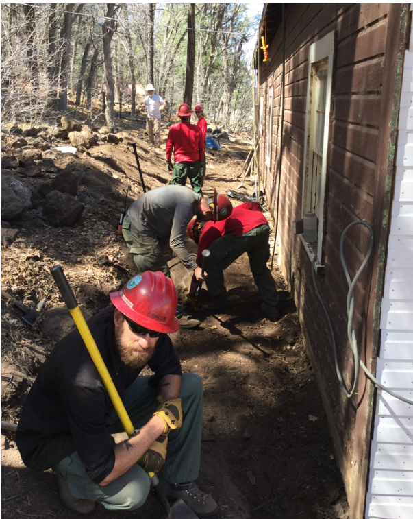
Members of the Mormon Lake Hot Shots volunteered time to help fix the drainage surrounding Mormon Lake Ranger House. (Jeremy Haines)
