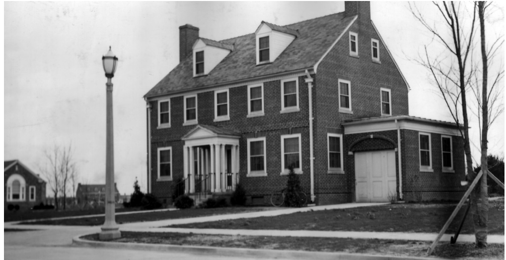
Noncommissioned officers' quarters duplex, inter-war housing at Fort Knox, KY, circa 1940 (NARA)
