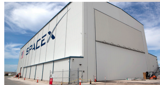
SpaceX built a horizontal processing facility at the base of LC-39A where it will process rockets and spacecraft before they are transported to the pad for launch. (NASA/Dimitri Gerondidakis)
