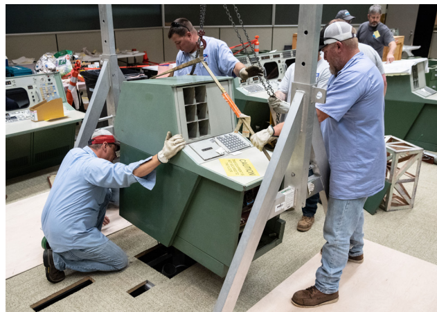
Installation of reproduced equipment. (NASA Johnson)
