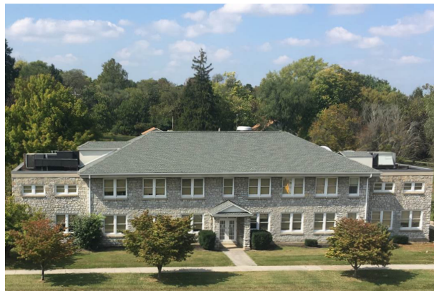
Front elevation of Leetown Administration Building (USGS)
