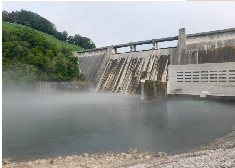
Norris Dam, TN (TVA)
