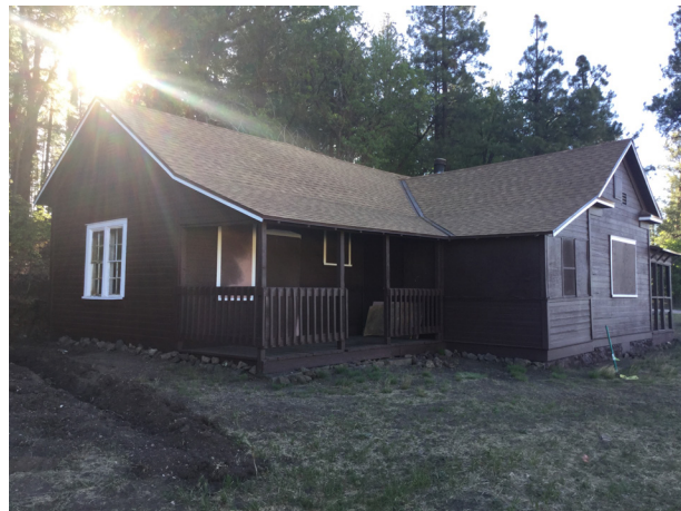
Mormon Lake Ranger House after rehabilitation (Jeremy Haines)
