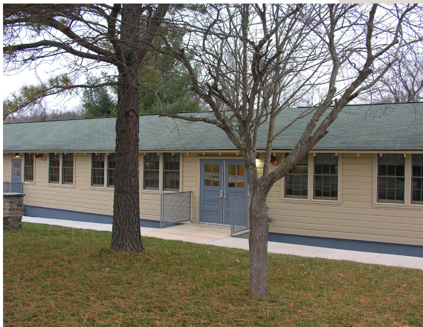
Countee Hall post-rehabilitation (U.S.Army)
