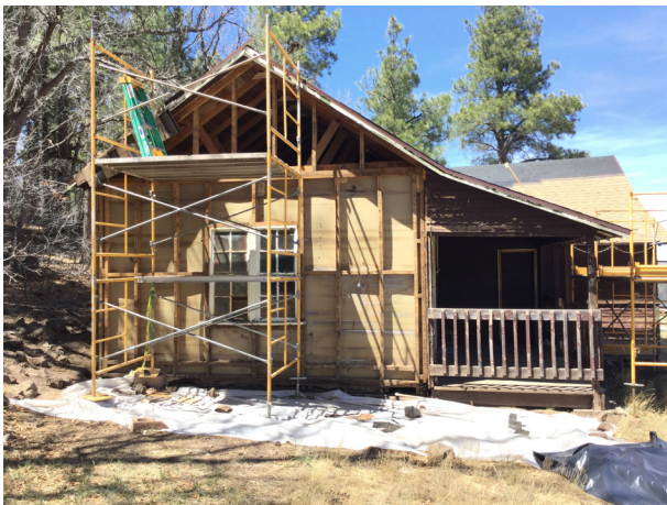
Mormon Lake Ranger House under rehabilitation (Jeremy Haines)
