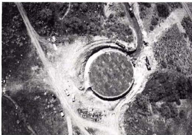
Water storage tank, Pleasant Grove, Utah. Plywood forming in place prior to pouring top of tank.
