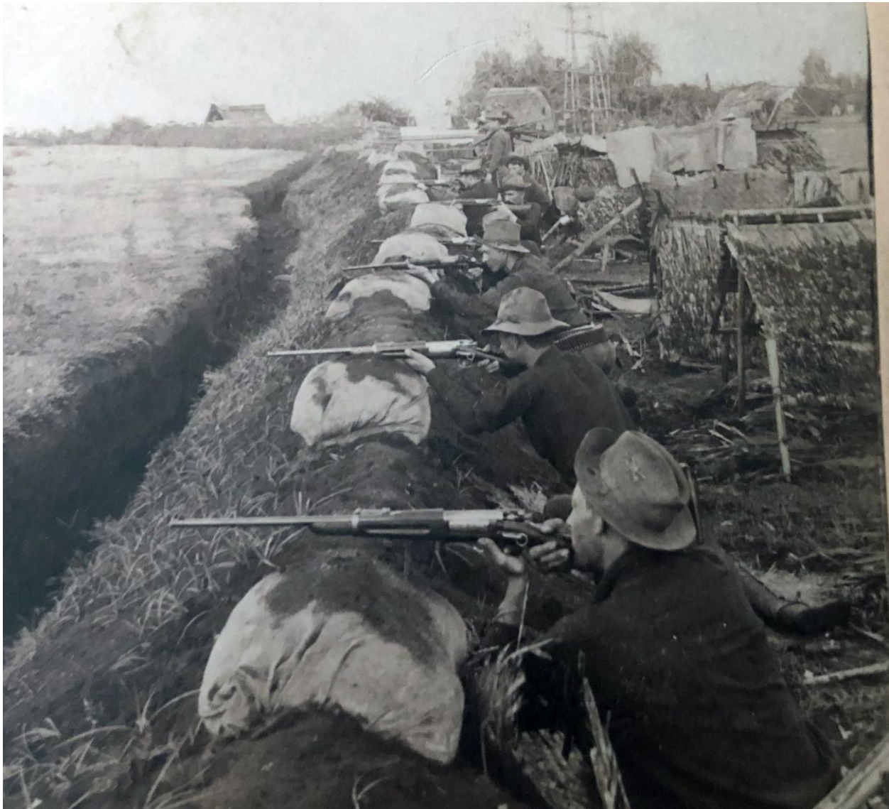
Figure 14. South Dakota volunteers use a prepared earth berm or parapet with a trench to the front for defense in the Philippine War. From a Works Studio stereograph, 1899.
