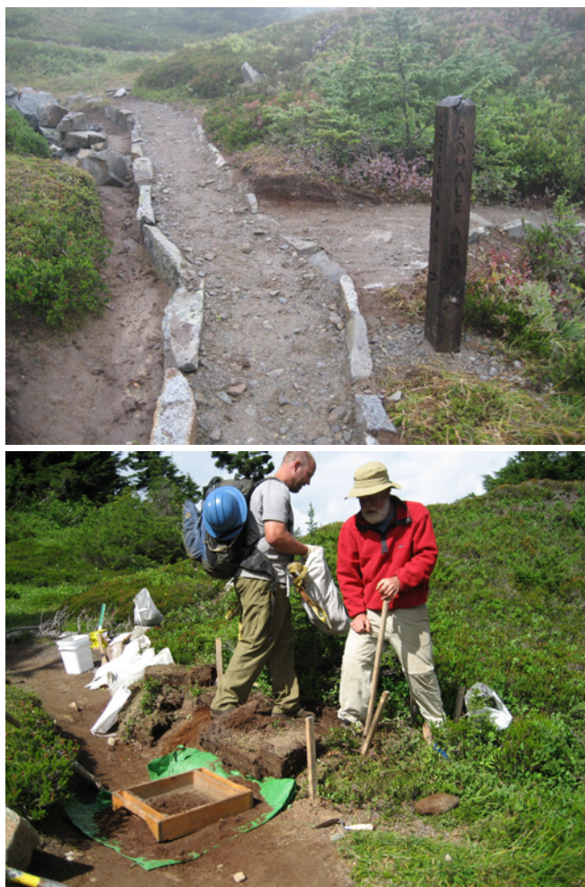
FIGURE 9. Lower image: stabilization of soil and hiking surface covering the Cascade Pass archaeological site, North Cascades National Park by Park Trails maintenance staff; Upper image: finished, raised section of hiking trail at Cascade Pass (images courtesy of Robert R. Mierendorf, 2008)
