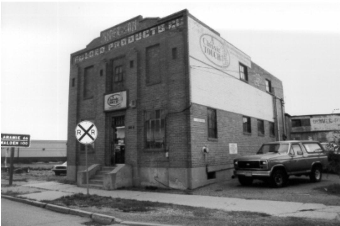
Figure 4. 300 N. College Avenue (5LR1502), looking northeast.
