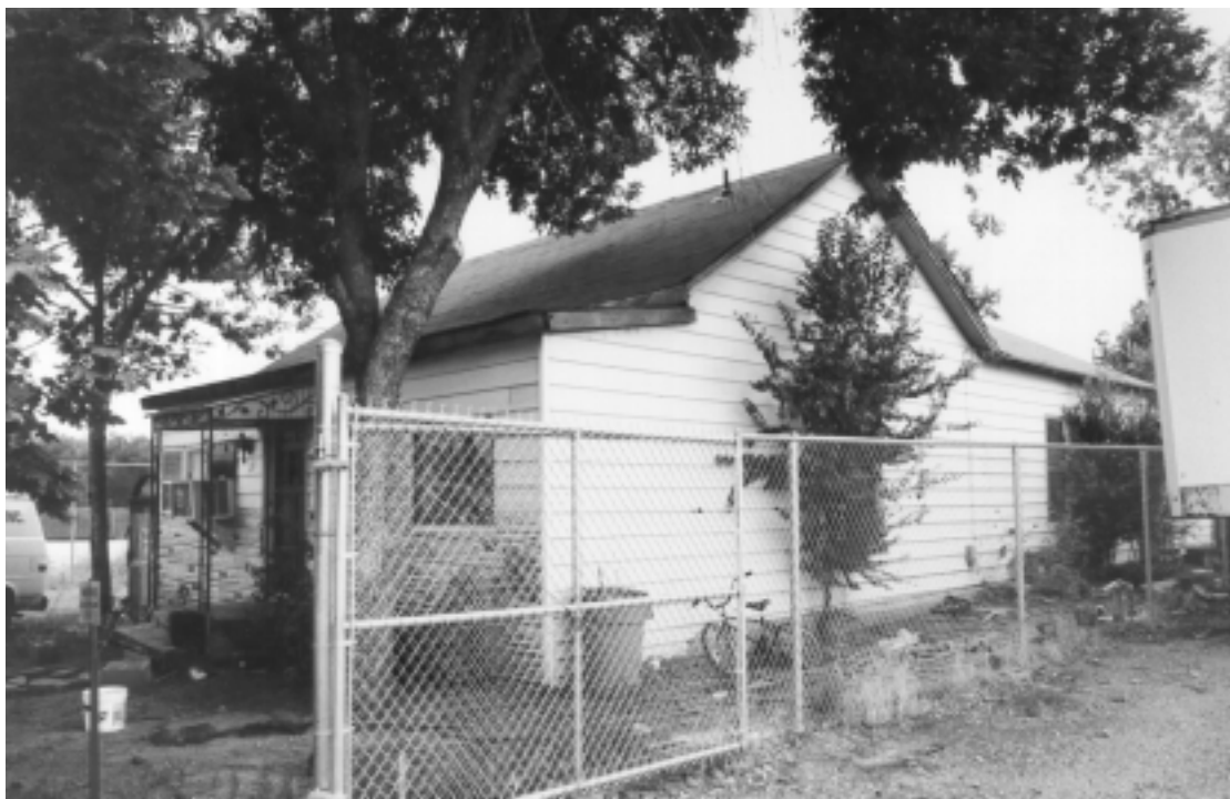
Figure 26. 414 Pine Street (5LR10311), looking east.
