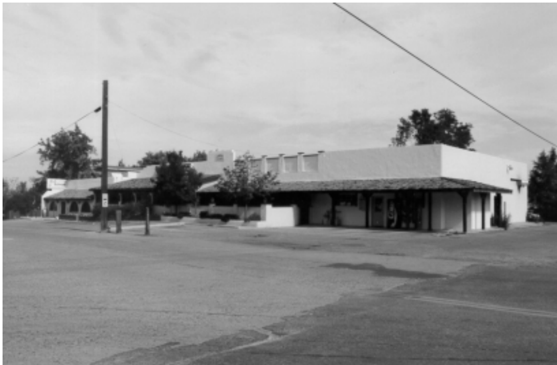
Figure 19. 400-404 Linden Street (5LR10306), looking east.
