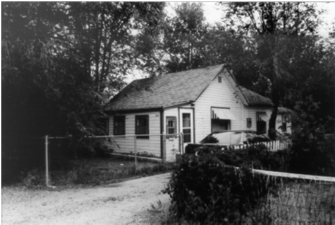
Figure 36. 226 Willow Street (5LR10320), looking north.
