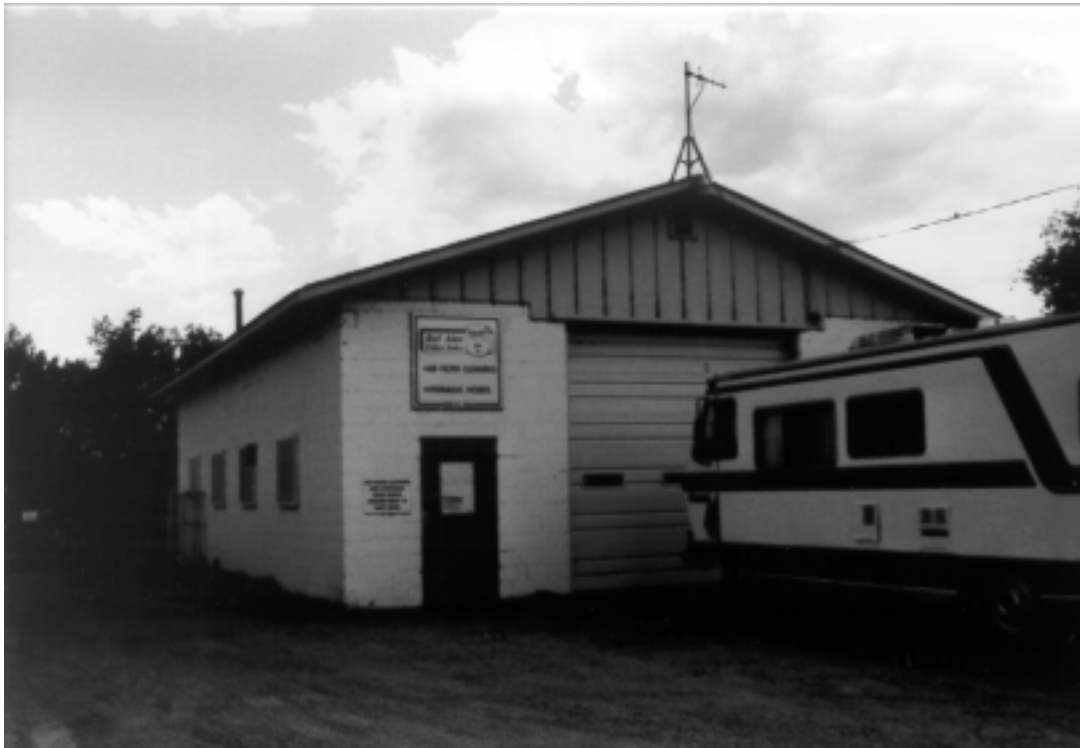
Figure 31. 203 E. Vine Street (5LR10316), looking south-southwest.
