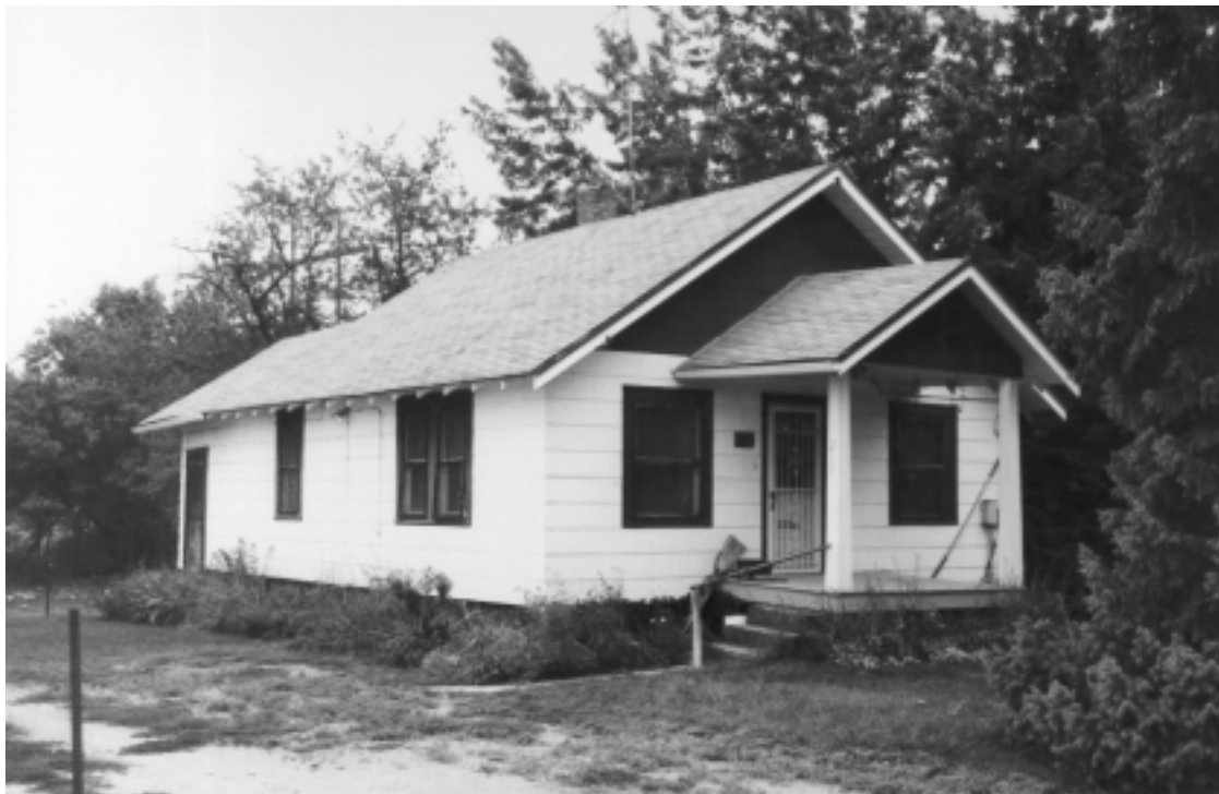
Figure 33. 213 E. Vine Street (5LR10318), looking southwest.
