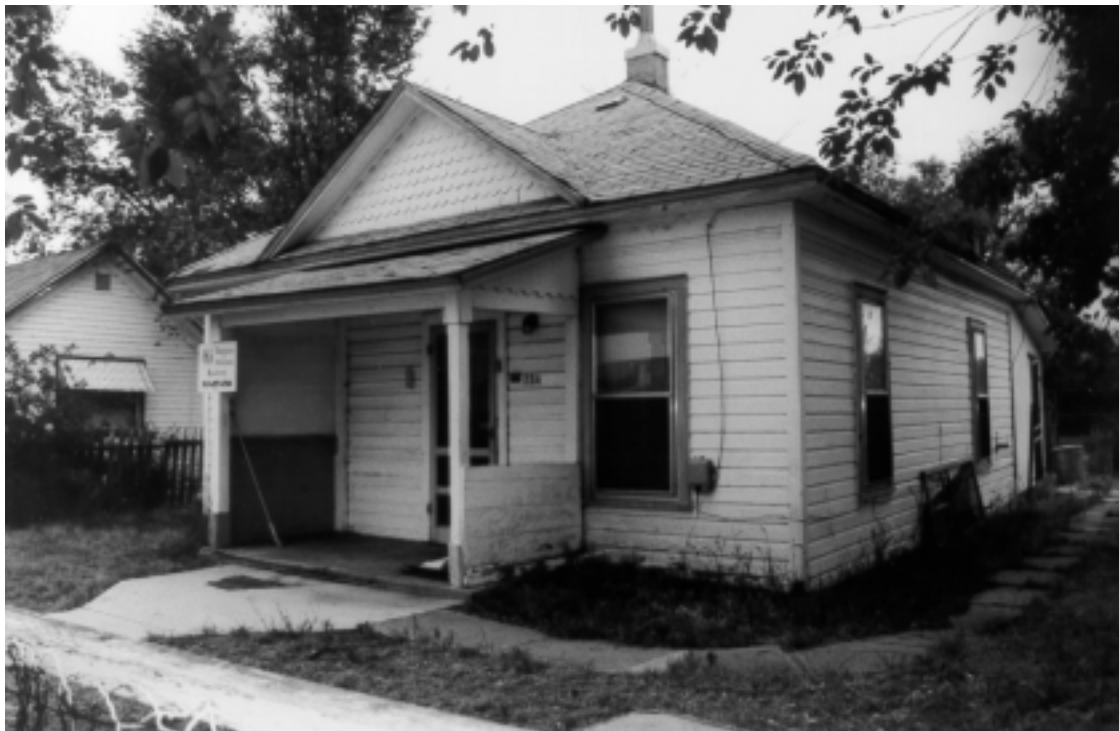
Figure 35. 224 Willow Street (5LR10319), looking north.
