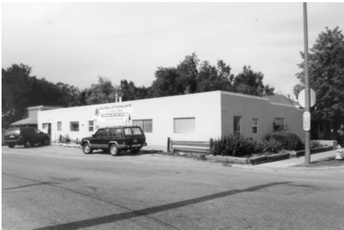
Figure 20. 401 Linden Street (5LR10307), looking north.
