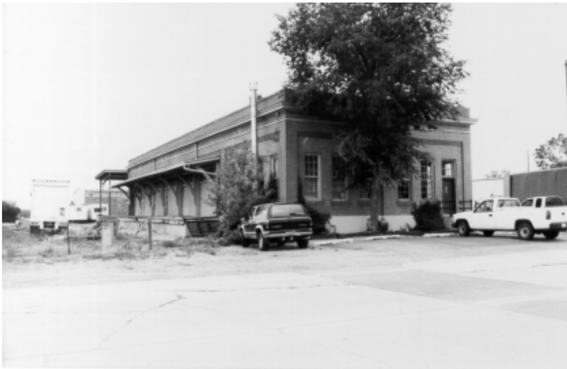
Figure 17. 350 Linden Street (5LR462.19), looking south.
