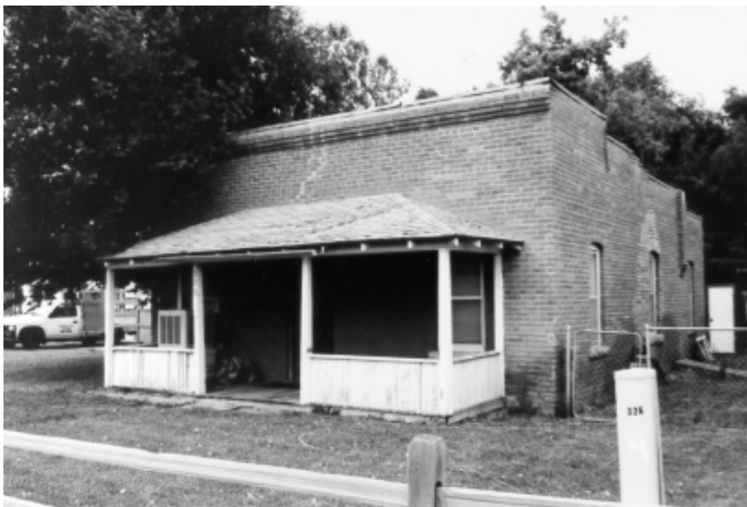
Figure 39. 326 Willow Street (5LR1562), looking north.
