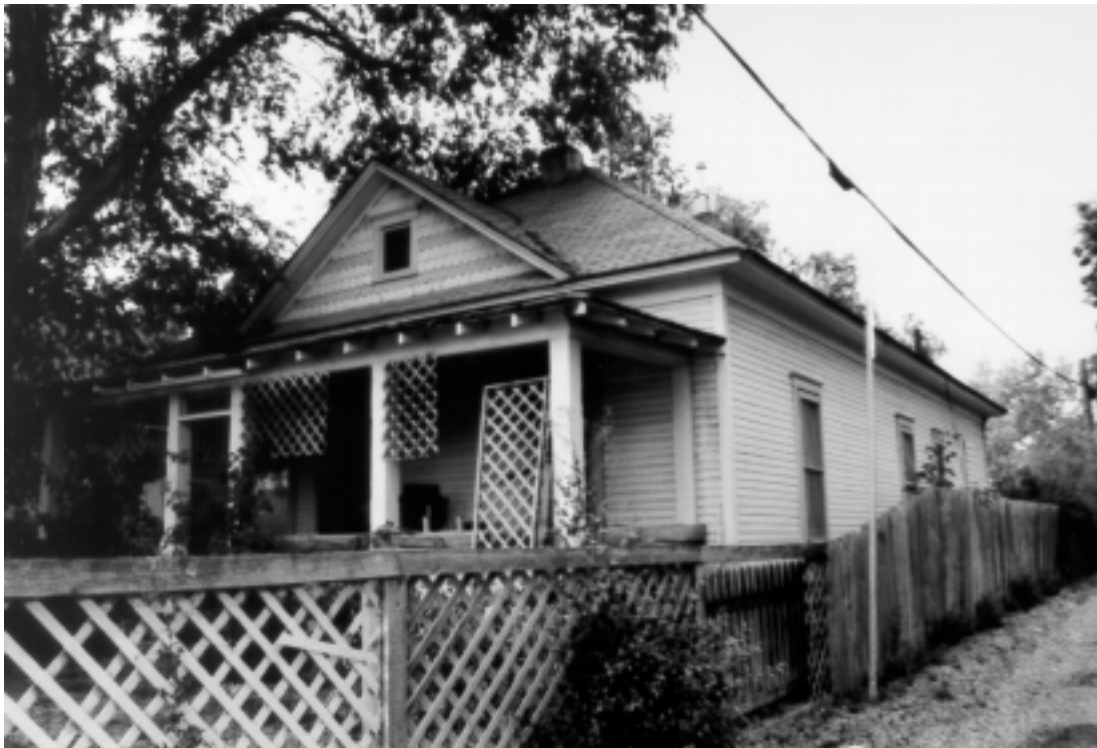
Figure 23. 409 Linden Street (5LR10354), looking west.
