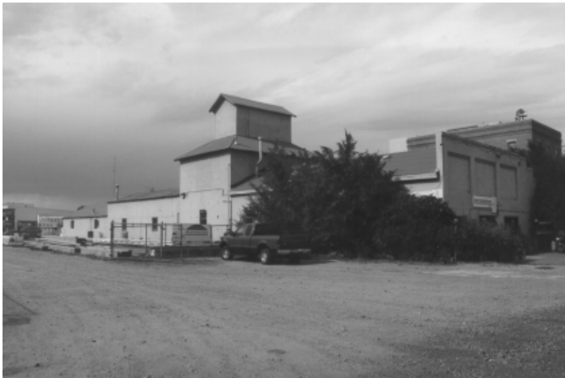
Figure 15. 119 Lincoln Avenue (5LR1900), looking north.
