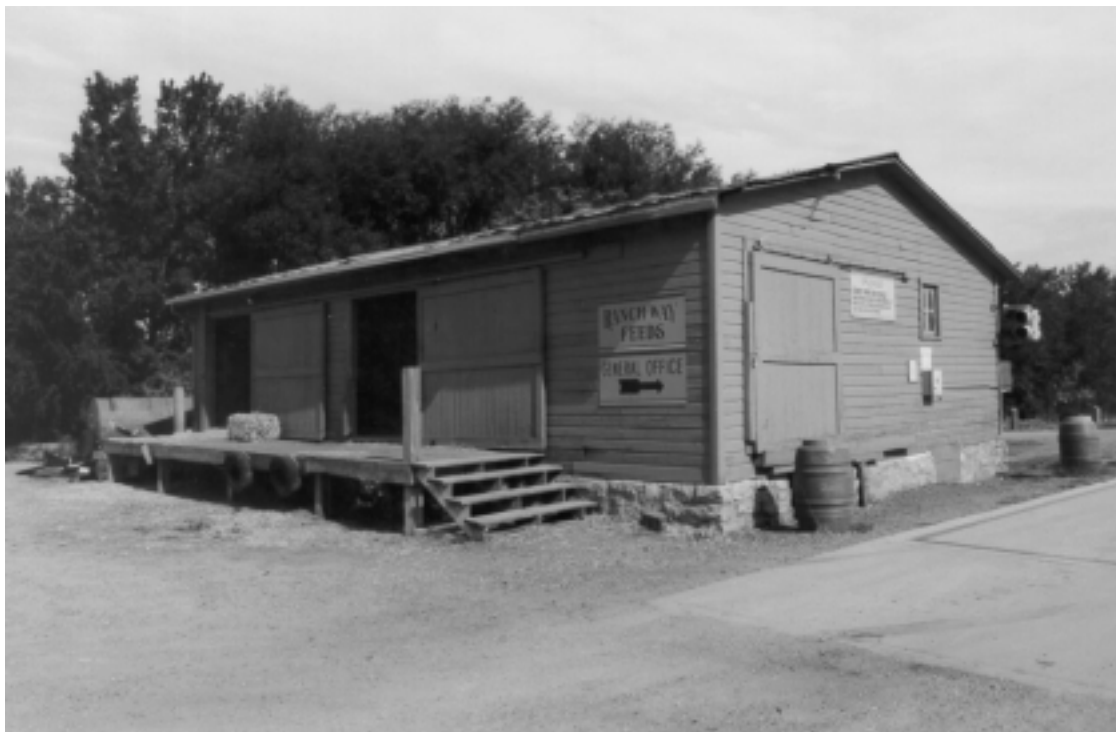
Figure 24. 416 Linden Street (5LR10309), looking east.
