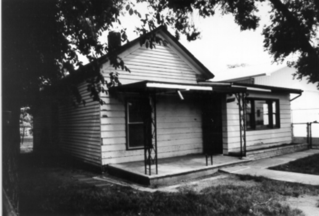
Figure 37. 308 Willow Street (5LR10321), looking east.
