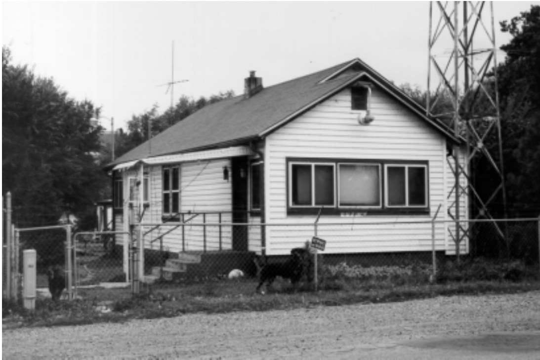
Figure 27. 101 E. Vine Street (5LR10313), looking southwest.
