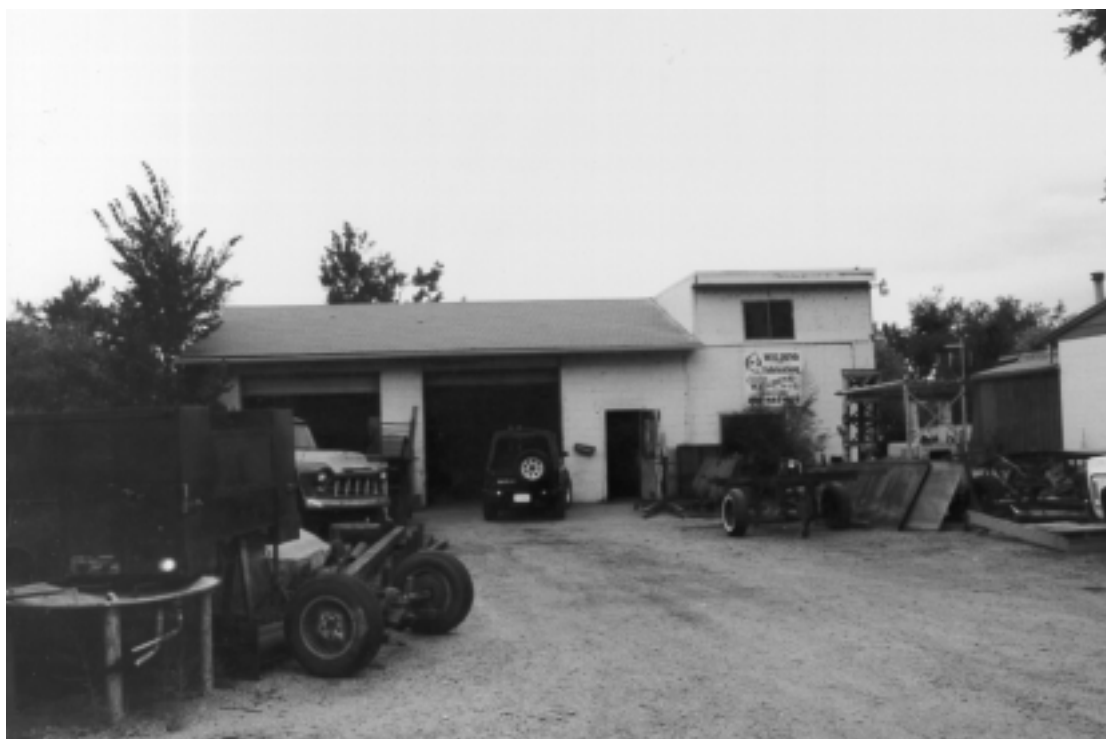
Figure 32. 209 E. Vine Street (5LR10317), looking south.
