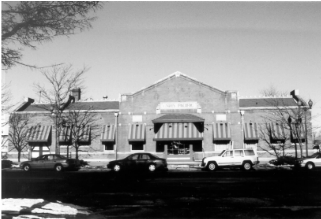
Figure 8. The Union Pacific passenger depot, 200 Jefferson Street (5LR462.12), view looking northeast.
