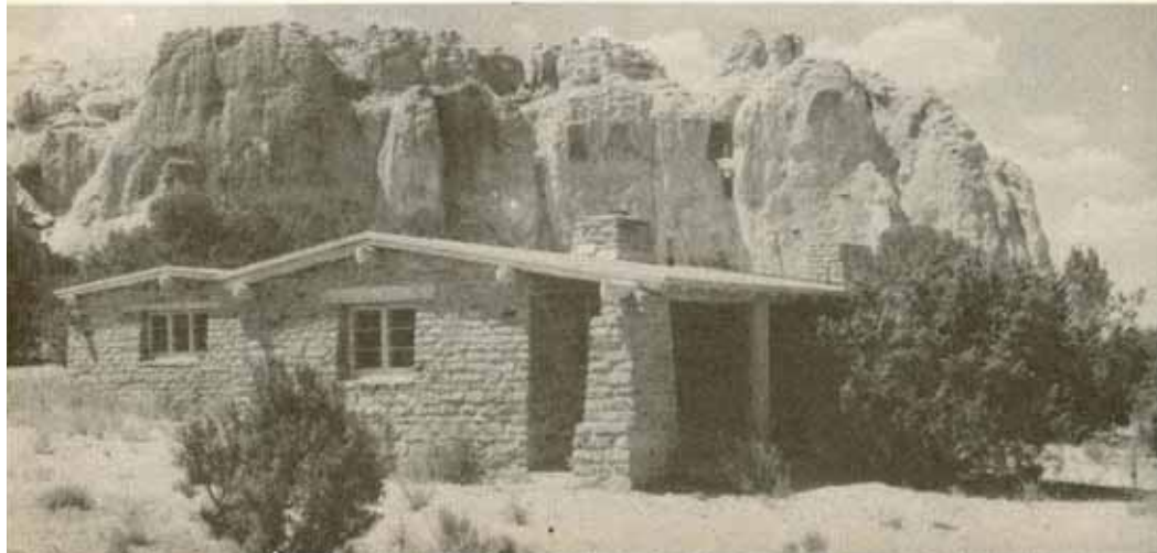
Custodian's office and residence
