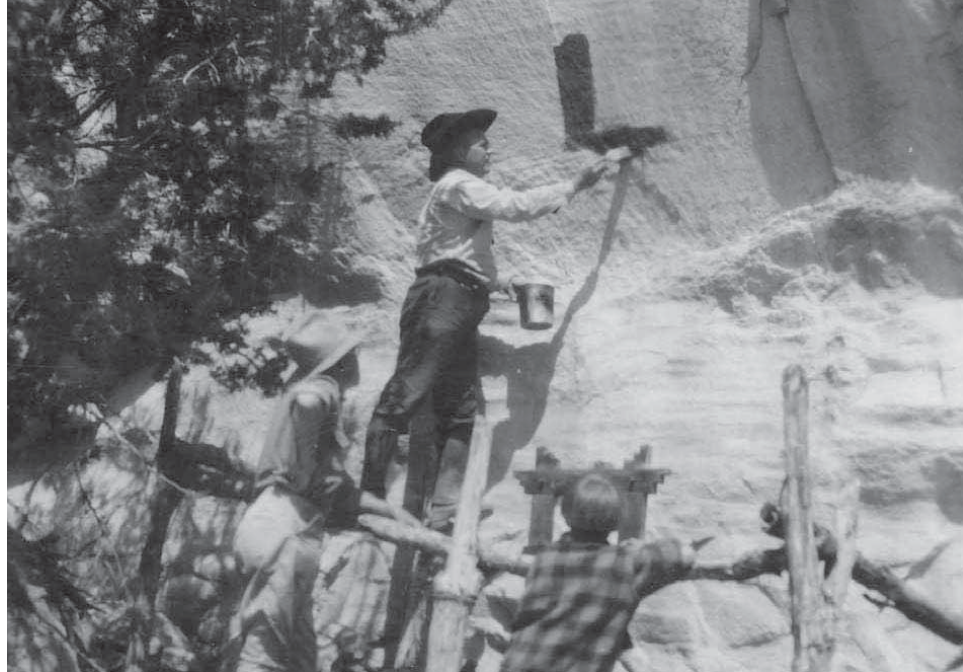
Figure 4.5: Vogt coating inscriptions along the trail with consolidants. Source: Vogt Photos, El Morro Archives, n.d.
