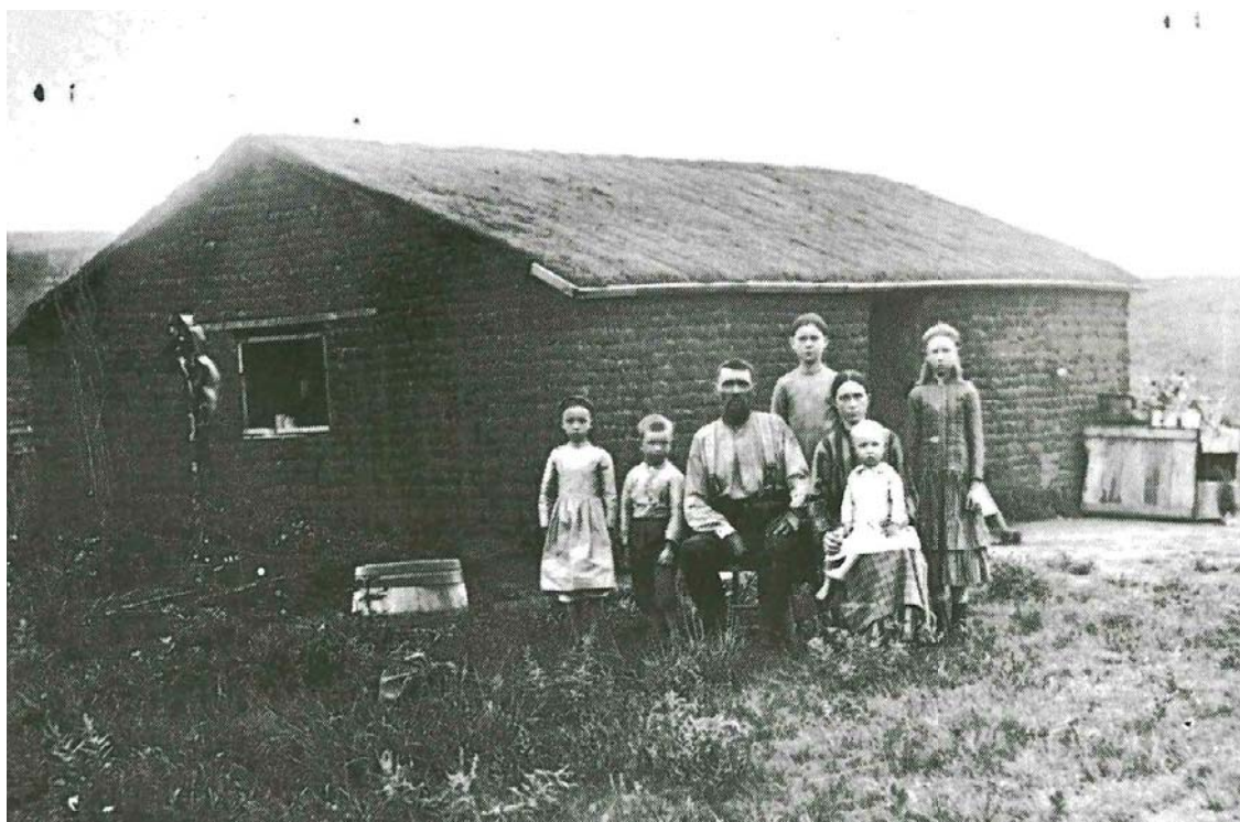
Figure 4.11. Example of a sod house in Nebraska. The barrel sunk into the ground near the corner of the house was a cistern (Welsch 1968:114).
