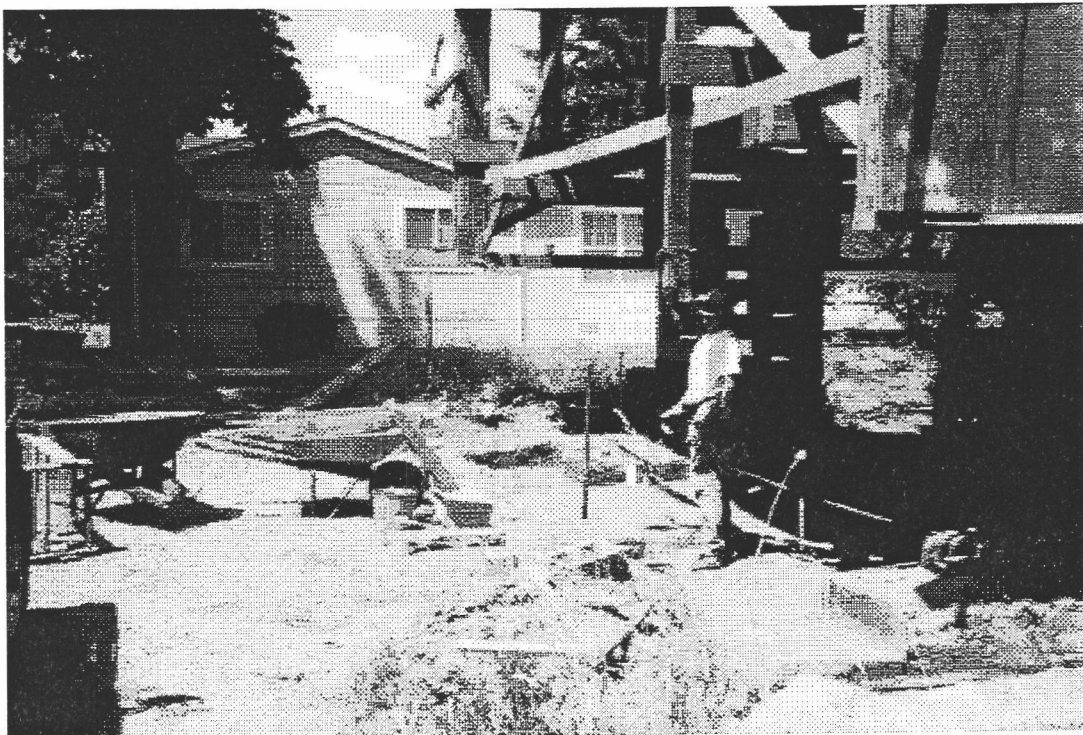
Figure 3.12 Foundation Trench Excavation (Research photo on file at Oregon State University)
