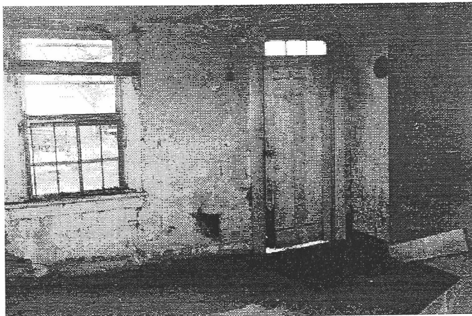
Figure 3.3 1993 Photo of Entry Interior (Research photo on file at Oregon State University)
