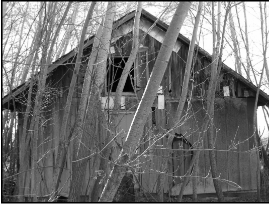
Historic Building Looking East at the North Elevation.
