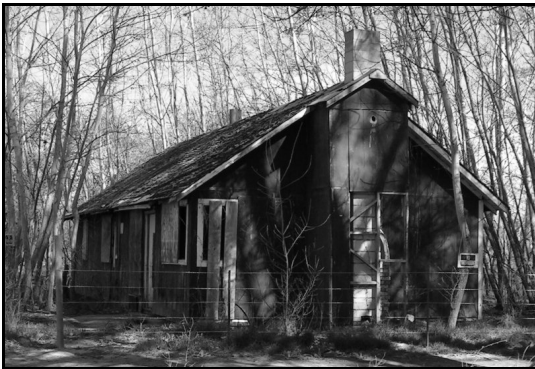
Historic Building Looking Northwest at the South and East Elevations.
