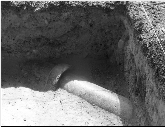
Figure 14. Drain Pipe Connecting to Southeast Corner of Foundation.
