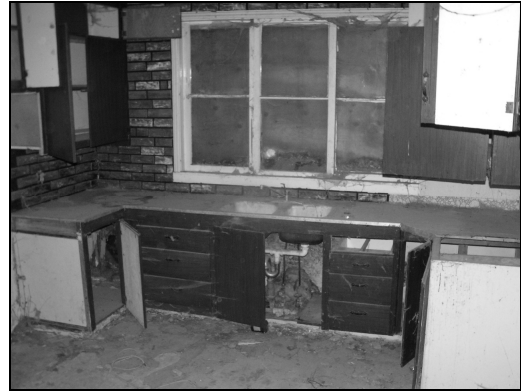
Figure 9. Interior View of Kitchen Area.
