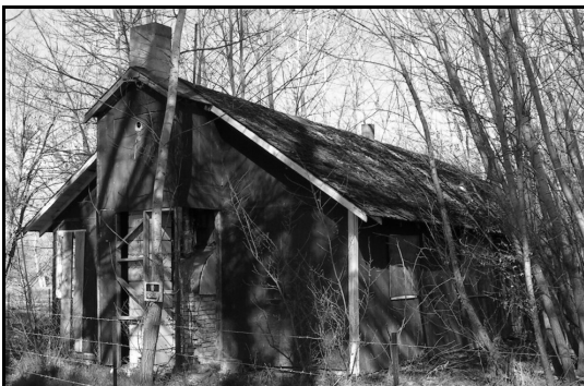
Historic Building Looking Southwest at the North and East Elevations.
