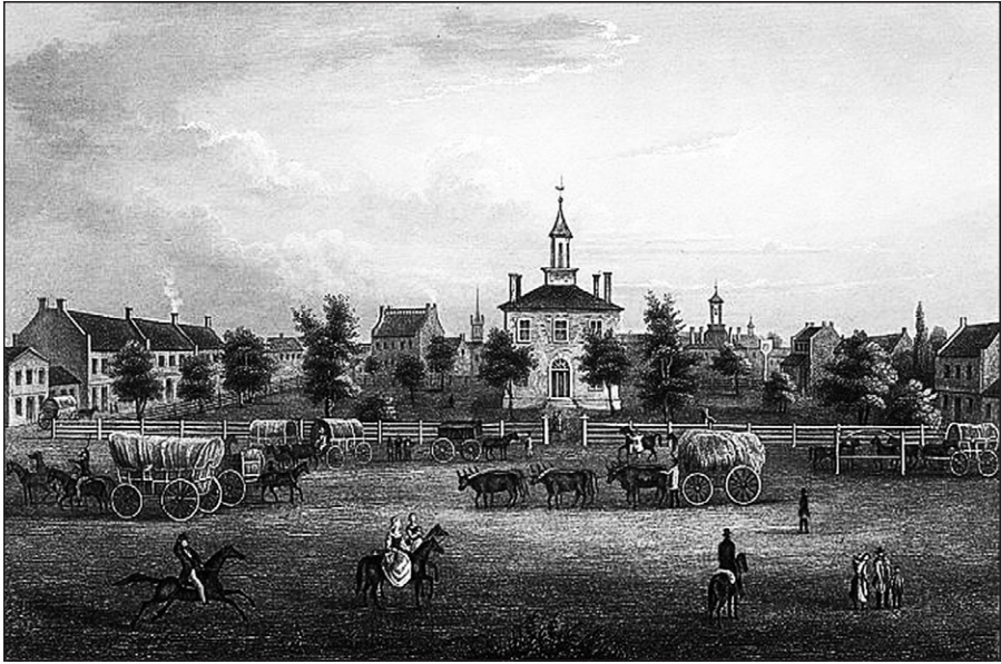
Figure 2.2. Hermann Meyer, Independence Courthouse, Missouri [1838], engraving, ca. 1850, Jackson County (MO) Historical Society Archives, JCHS4862L.
