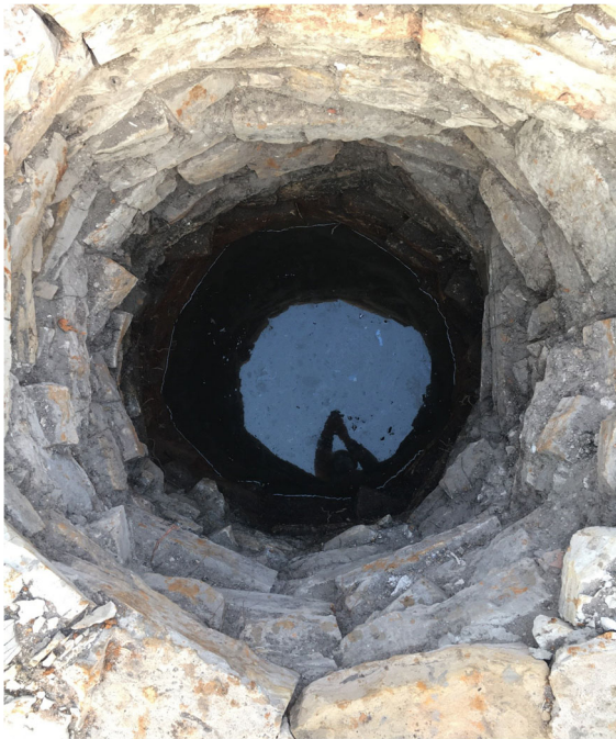
Fig. 5 The well in the Carter Complex (“Sutler’s Premises”) after excavation. The walls are made from limestone, and the conical-shaped well flairs outward at the bottom, making the bottom wider than the top. (Photo by A. Dudley Gardner, 2020.)
