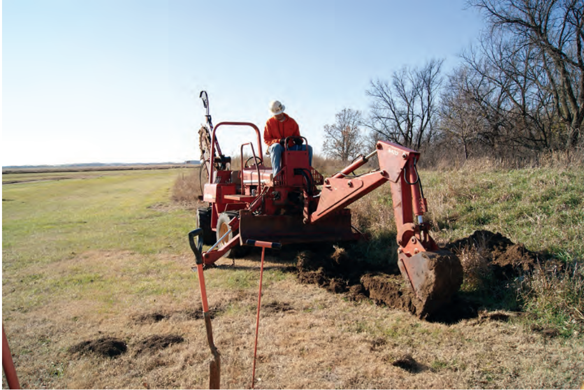
Figure 17. Excavation of access pit 1 with a backhoe (view to the southwest).
