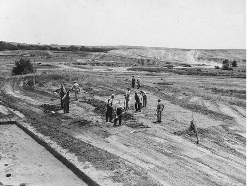
9.1. Workers excavating at House 5, 25FT13. Initial phases of dam construction are in progress in the background.
