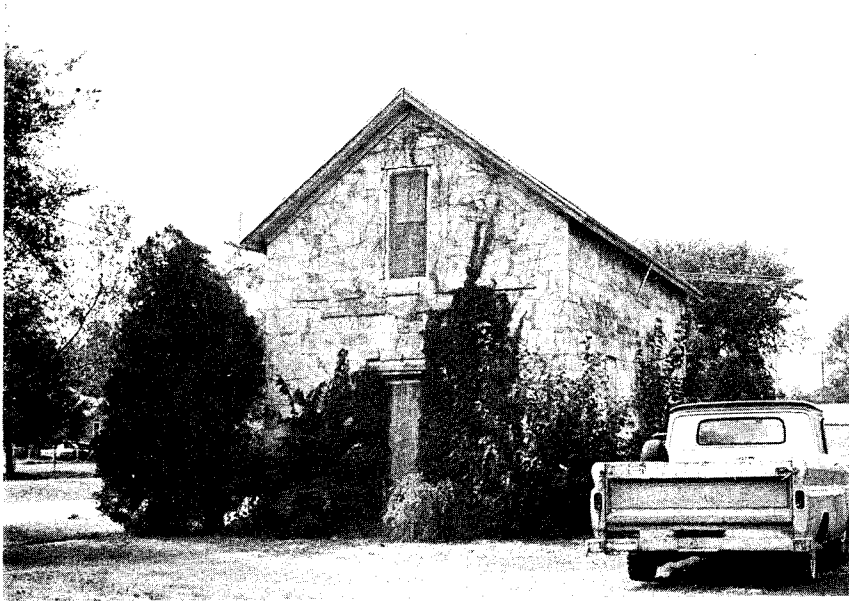
A: Stone House, Within Zone of Potential Significance (EN-Z1), Enterprise, Dickinson County
