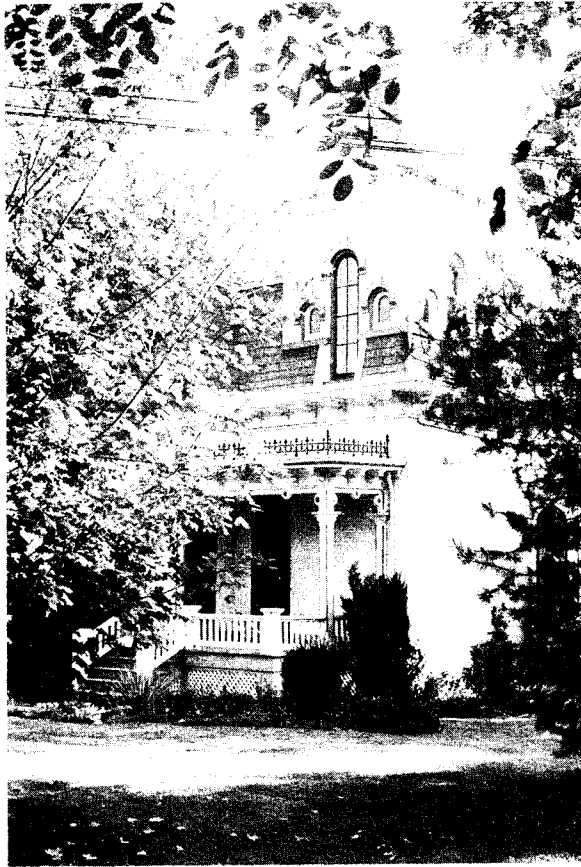
A: Corner Tower Detail House Within Zone of Potential Significance (LW-Z1) Lawrence, Douglas County
