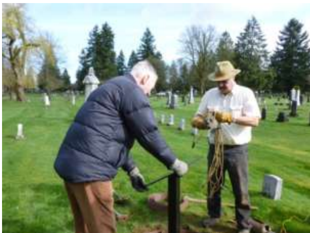
Bob Kabel supports Nathan's plaque while Chuck Hornbuckle prepares rope to temporarily secure the marker while pouring the concrete base.
