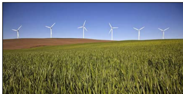
The Biglow Canyon wind farm near The Dalles
